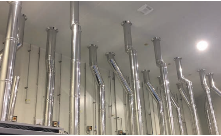
10 bakery ovens, 8 roll on ovens 2 Multi-purpose cookers Ø 250mm
